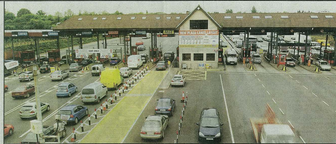
West-Link toll bridge: an example of a successful public-private partnership in action
